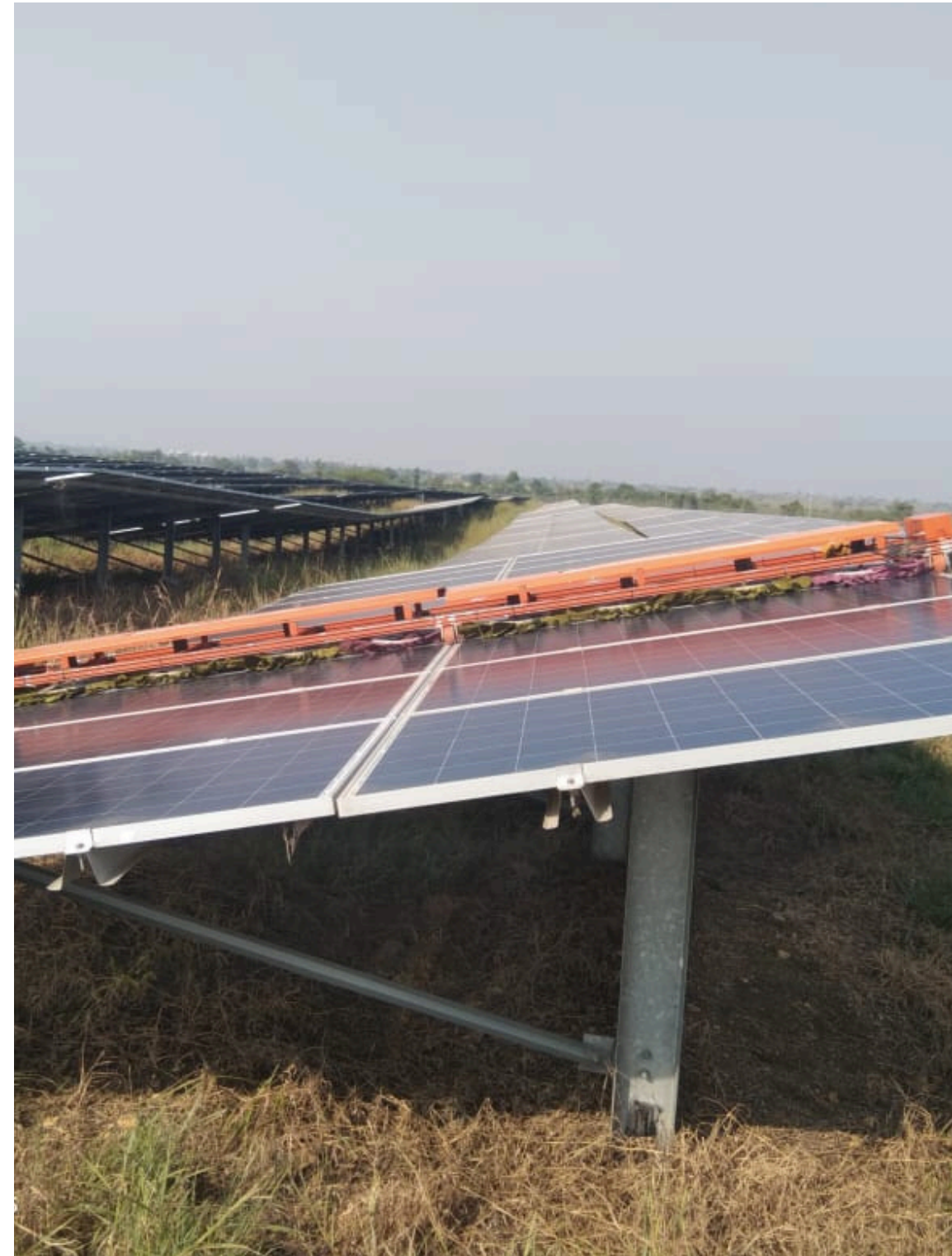
Module Cleaning under progress
